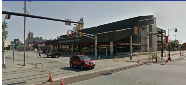
EXISTING: Walter Rand Transportation Center
