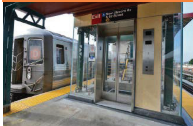
PROPOSED: Platform Elevator
